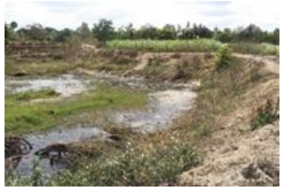
2. Desilting of Tank at Bitravalli
